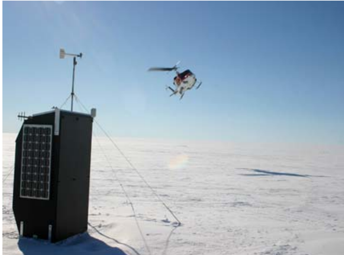
Mobile Base Station at SANAE, powered by PV and wind energy
