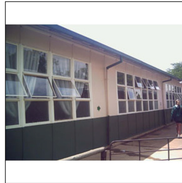
◀ Northern facade at a pre - fab building. ▶
